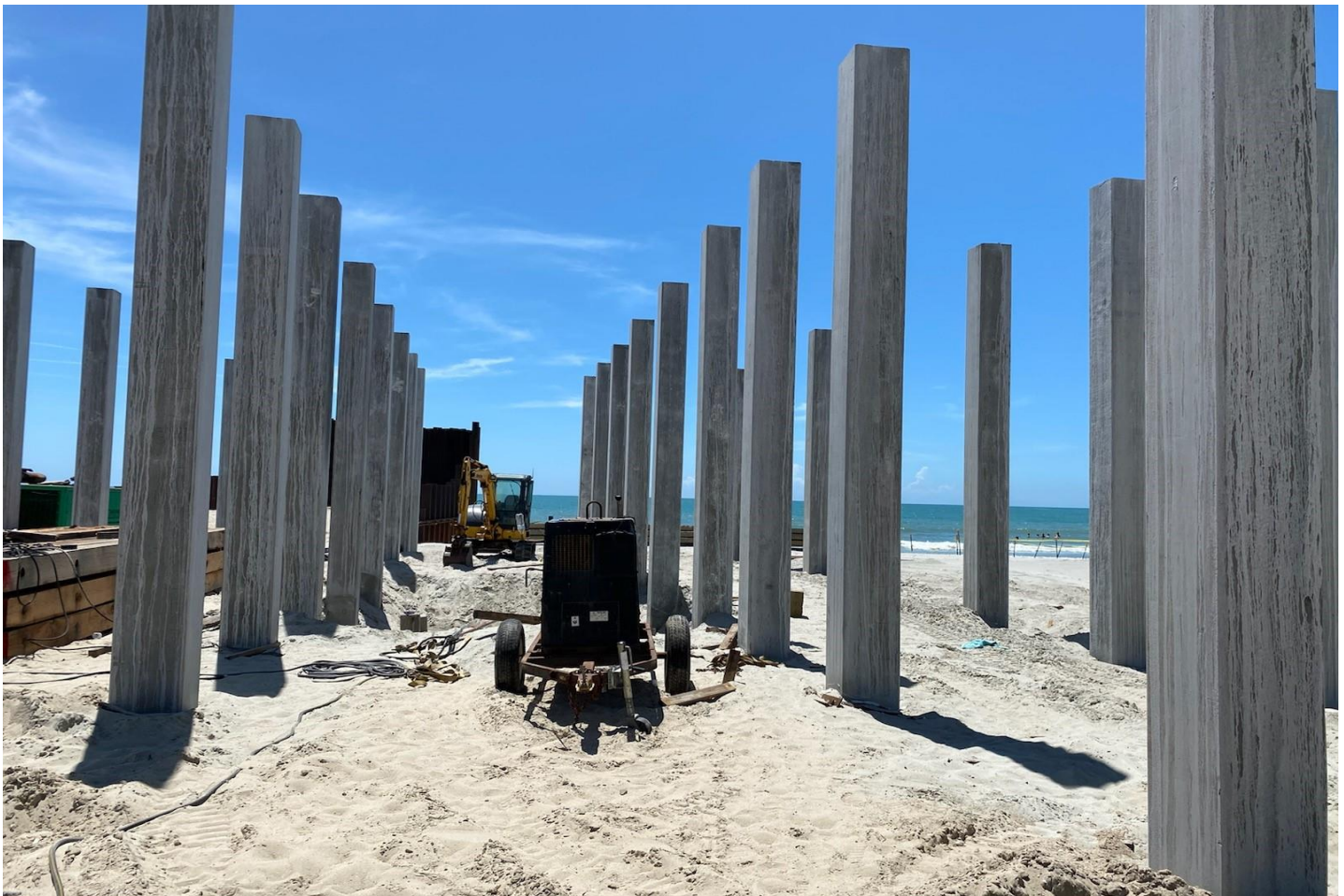
Pier podium piles continue to be installed 6-30-21
