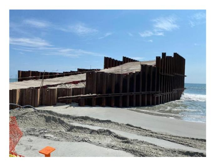
The trestle ramp, which will be used as a work platform to construct the ocean pier, is substantially complete and ready for the large crane.
