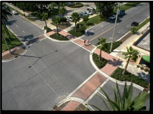
Example of an intersection with well-defined crosswalks. This traffic calming technique signals to motorists that they are approaching an area with regular pedestrian traffic.
