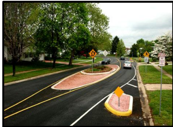
Example of a roadway that has been narrowed to discourage speeding.
