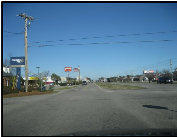
US 17 Business frontage road looking north from Glens Bay Road.
