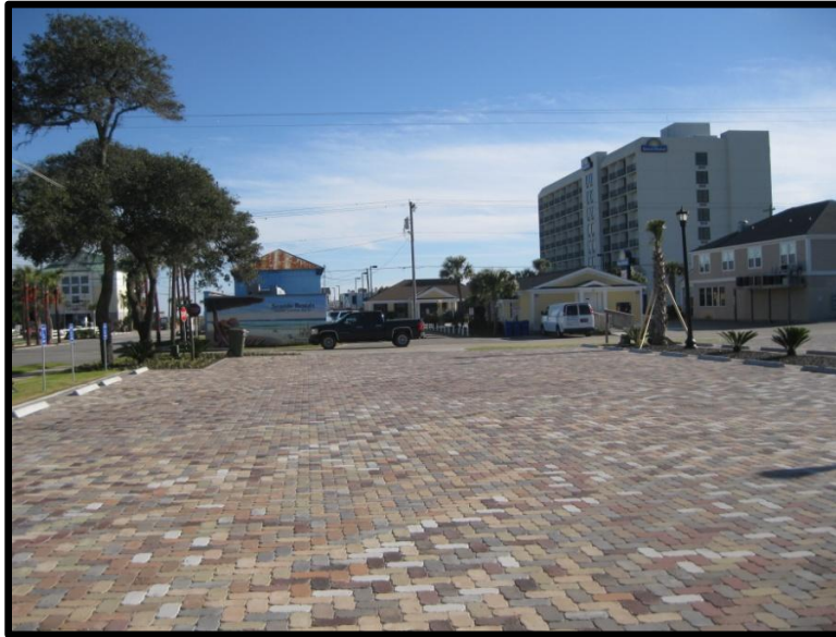
Yaupon Drive Parking Lot
